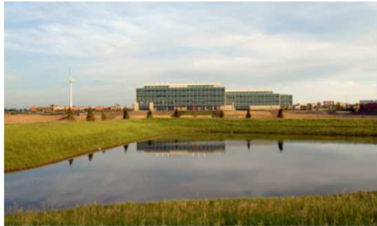
Arbor Lake, located just north of Great River Energy headquarters made the building's innovative lake-source geothermal system possible.
