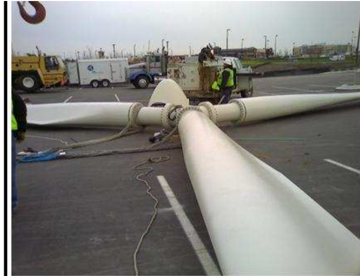
Crews assemble the wind turbine rotor and prepare to hoist it to the top of the turbine.
