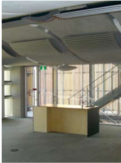
Wavy concrete ceilings provide thermal mass to stabilise internal temperatures.
