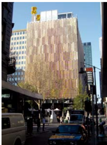
Swanston St façade with adjustable timber louvres to screen westerly sun.
