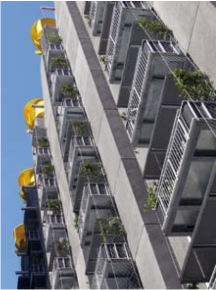
Vertical gardens run the full height of the northern façade assisting with shading, glare and air quality.
