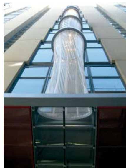
CH2 has five shower towers visible from the street that shower water down a 3.5 storey enclosure to cool air and water. The air is then used for the retail spaces.
