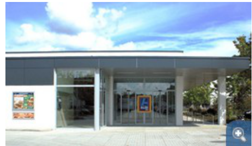
The new discount supermarket in Rastatt wants to be exemplary in terms of energy efficiency © Aldi Süd
