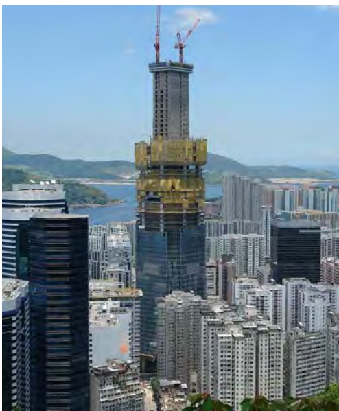
Figure 1: One Island East, Hong Kong (Gehry Technologies, 2009).
