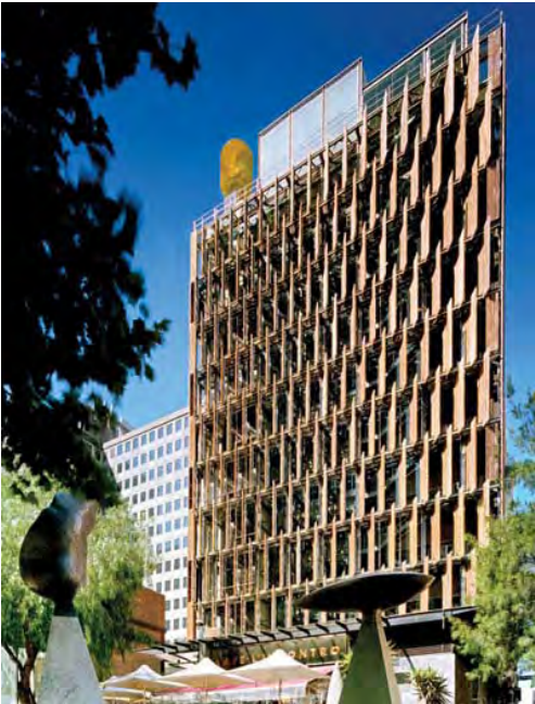
Figure 3: Council House 2, Melbourne (Fortmeyer, 2008).
