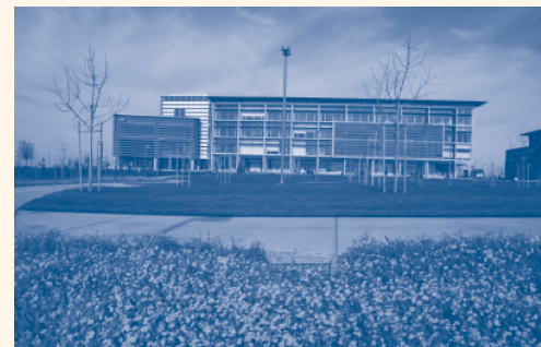
Figure 1: Pilot program shows MBCx savings Monitoring-based commissioning (MBCx) reduced building-energy consumption by identifying and correcting faulty system operation on California campuses.
