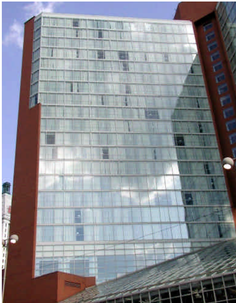
The Hyatt in Cincinnati – An all glass façade with occupants indicating their preference for solar control by drawing the interior shades
