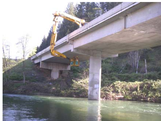
FIGURE 8 HydraPlatform Source: CH2M HILL
